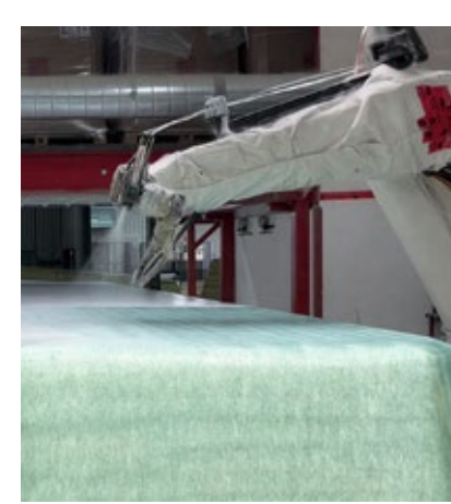
3 Barrier Coat Application
